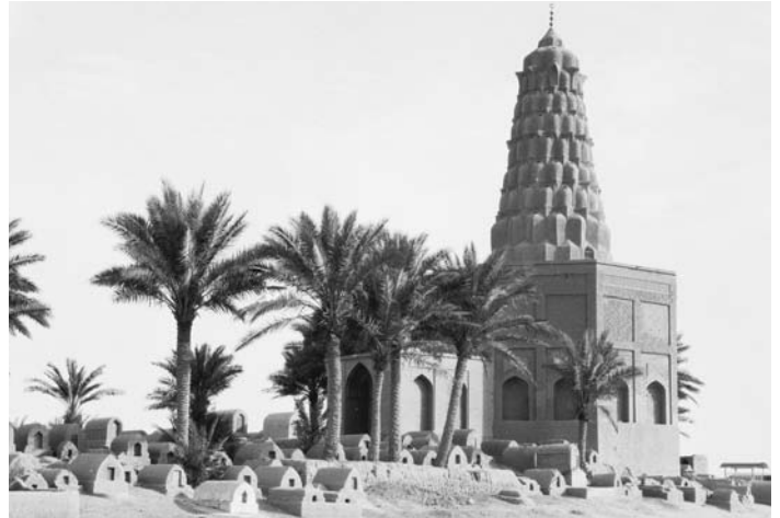
Sitt Zumurrud Khatun's tomb is the most famous mausoleum in Baghdad and was constructed before 1202.
